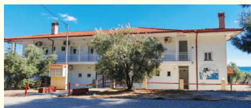
1. KUĆA ALEXANDRA GPS N40.259388/E23.490658
