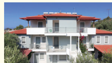
2. KUĆA ZEPPOS GARDEN GPS N40.045734/E23.814944
