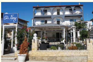
5. KUĆA FAY GPS N39.98934/E23.89796
